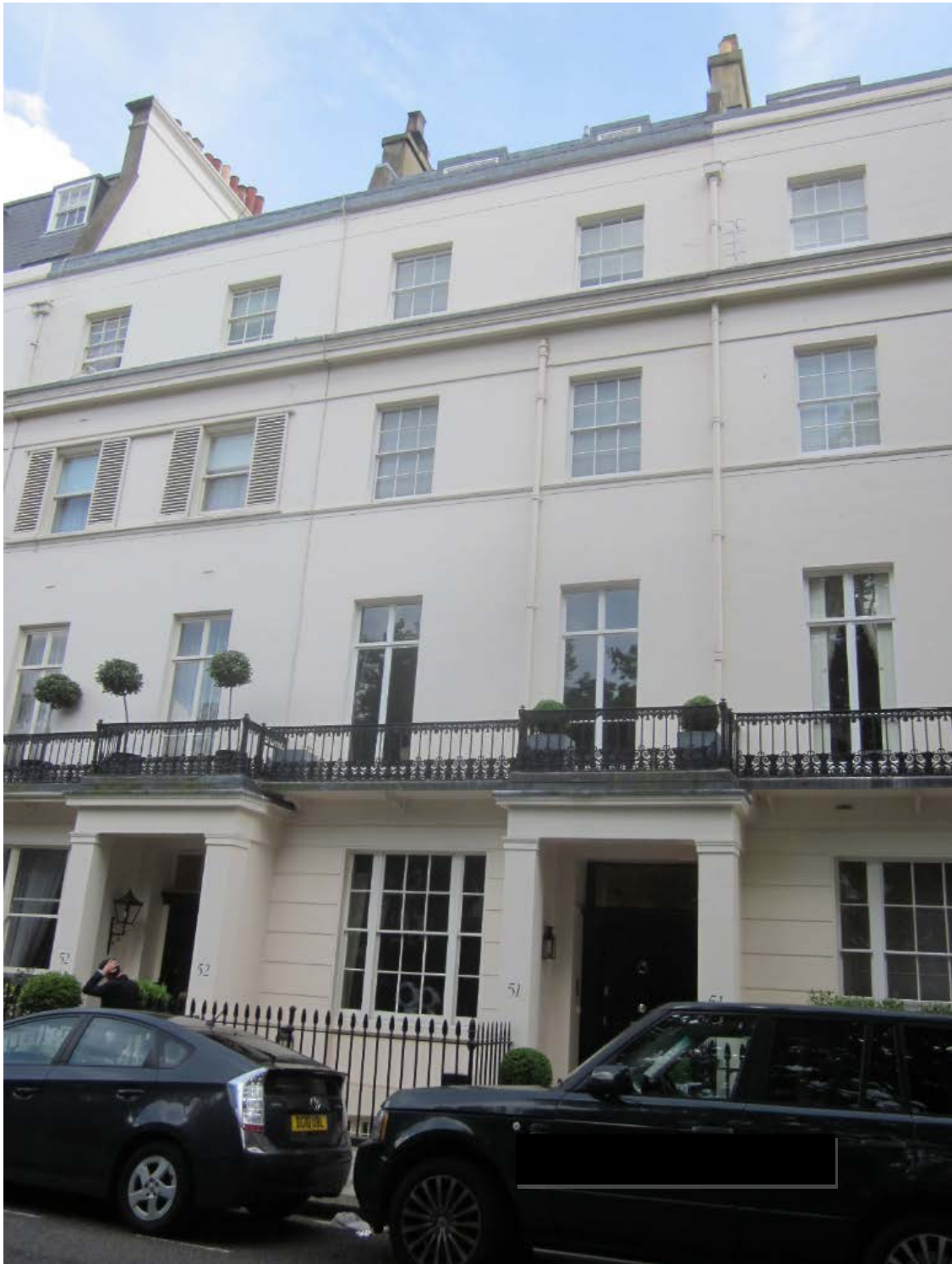
Front elevation of application property
